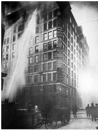
COURTESY: CORNELL UNIVERSITY Fire-enchanted sprinkler systems were considered too costly by many factory owners and were not installed in the Asch Building.
